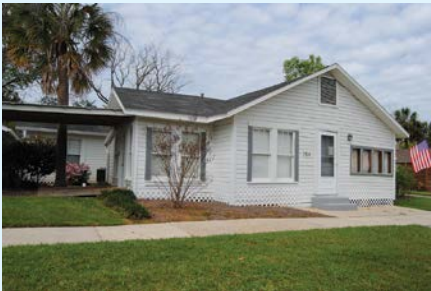
7 W.L. MERCHANT HOUSE (754 S. THIRD STREET)
